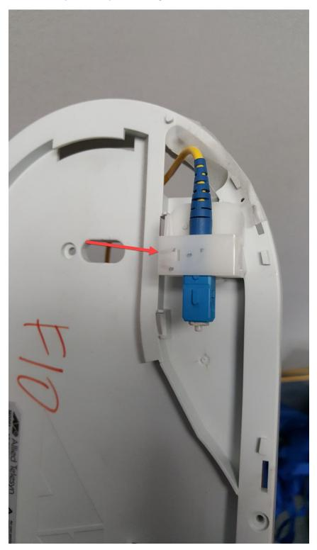
Once the top half of the clip is removed then the fiber cable should easily be able to be removed from the back plate and the tip of the cable pulled through the hole of the back plate. Feel free to dispose of both the back plate and wall mount once removed.
